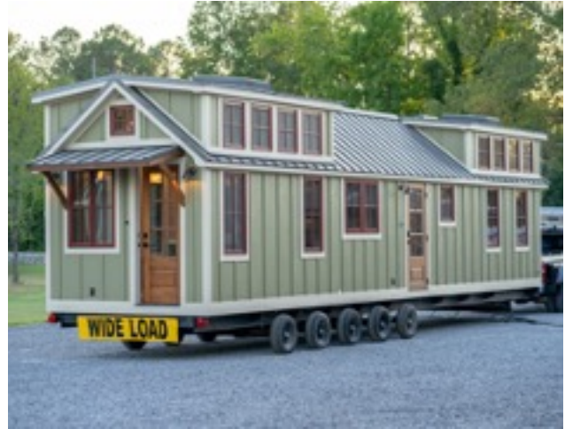
Manufactured tiny home – housing built off-site and shipped to its final location.
